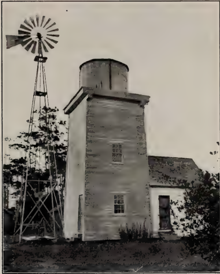
Fig. A. Wind-mill, pump and tank in a citrus grove.
